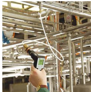
Control a dryer with DP 300
